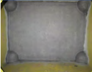
Container After Grit Blasting
